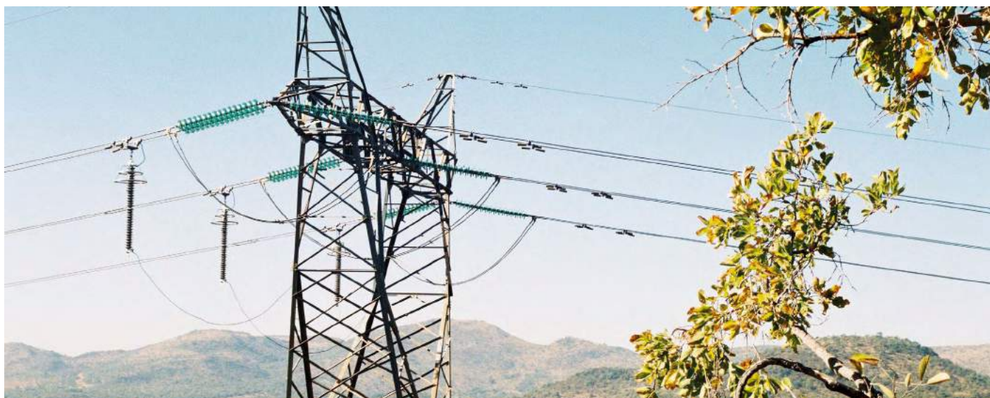
Line surge arresters, incorporating PEXLIM Q arresters and disconnecting devices on earth leads, erected on ESKOM 300 kV system in South Africa.
