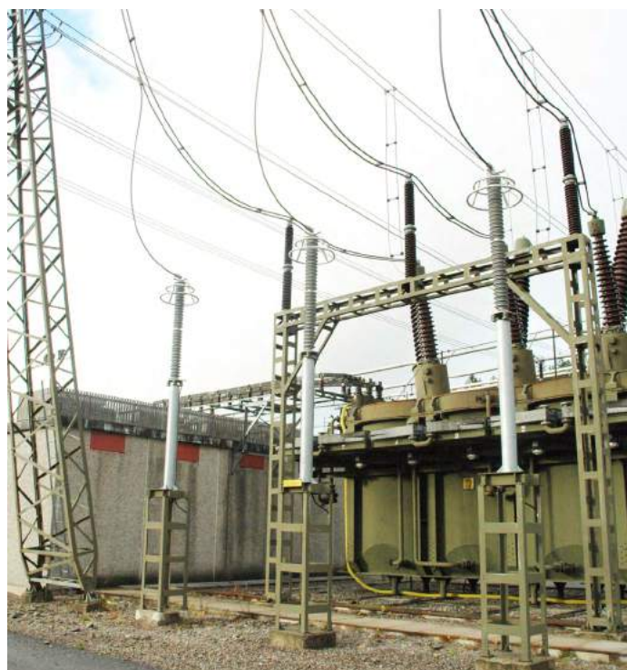
PEXLIM surge arresters protecting a 420 kV power transformer in Sweden
