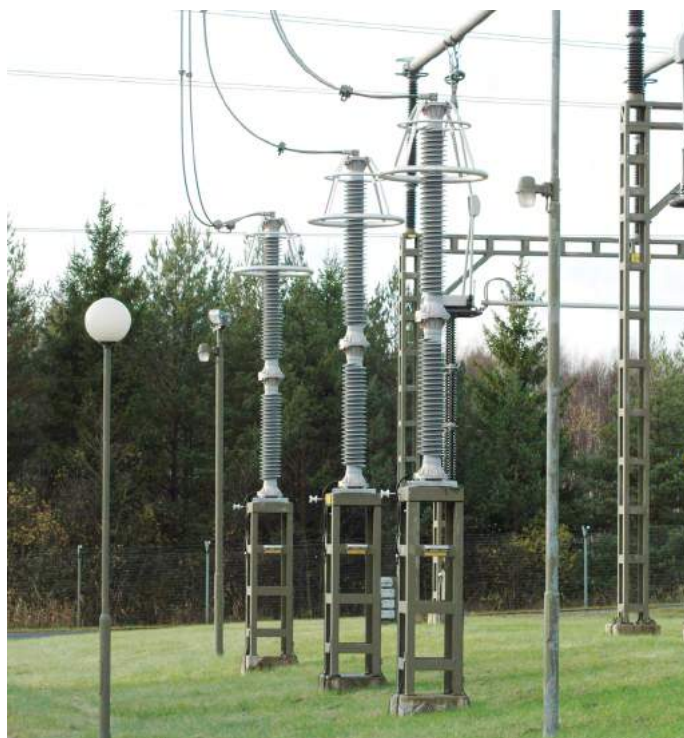
TEXLIM surge arresters connected to the line entrance
