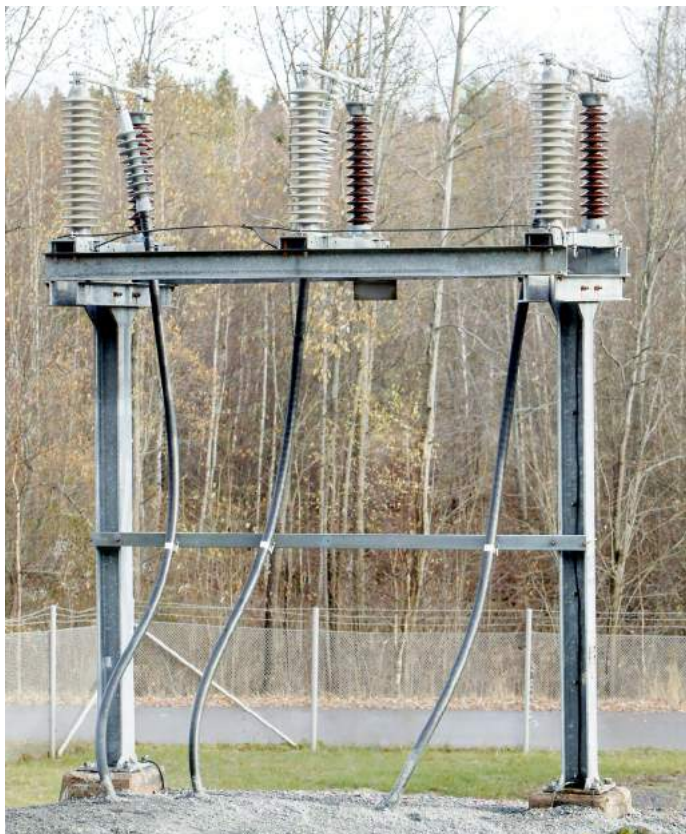
PEXLIM surge arresters protecting a cable entrance
