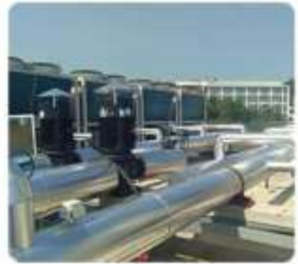
Power plant flue gas treatment
