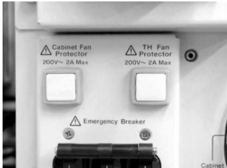
Figure 2-8 Fan protector switch for E3160-60065, E3160-60066, E3160-60067, and E3160-60068
