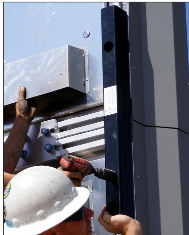
Figure 15: Aligning and Installing the Vertical Splice Tubes
