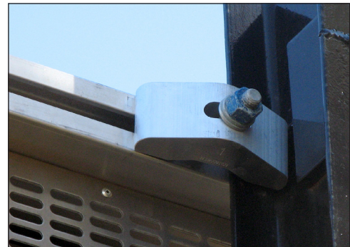
Figure 5: Rocker Clamp Engaging Upright
