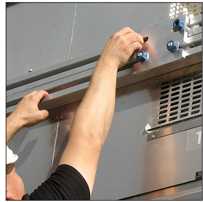
Figure 13: Attaching Splice Plate
