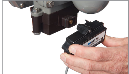
2. Press the activation module onto the sensor.
