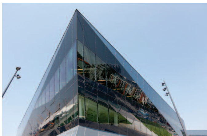
Situated at the heart of London's Green Enterprise District, the Crystal, a sustainable cities initiative by Siemens, will be an iconic landmark demonstrating Siemens' commitment to creating sustainable cities. The exciting new building will feature conference facilities, research space and an interactive exhibition.
