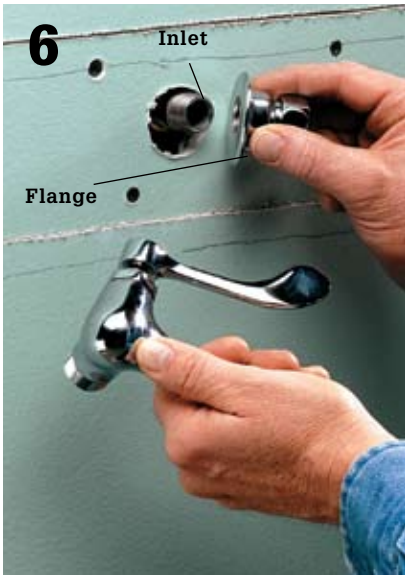
Cut and install the wallboard patch. Fit the flange over the inlet. Apply pipe joint compound to the threads of the faucet body. Assemble and adjust the faucet according to the manufacturer's instructions. Test the faucet before refinishing the wallboard.
