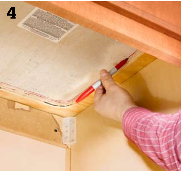
4 Install the tile underlayment. Granite tile, like ceramic tile, requires a cementboard or denseboard underlayment layer. Cut the material (see page 114) to the same dimension as the plywood subbase and lay the cementboard over the plywood with the edges flush. From inside the sink base, trace around the sink cutout with a marker. Remove the underlayment and make the cutout with a jigsaw.
