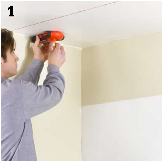
Mark the desired outline of the soffits onto the ceiling. Use a carpenter's square to mark square corners. Use a chalk line to mark long straight sections. Use a stud finder to locate the ceiling joists and the wall studs in the area of the soffits.
