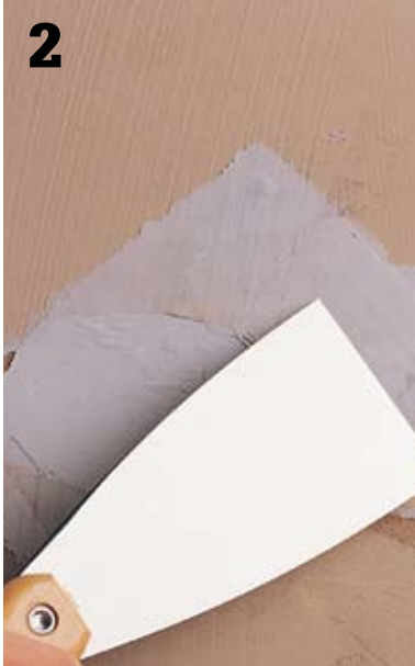
Apply spackle to the edges of the chipped paint with a putty knife or a flexible wallboard knife.
