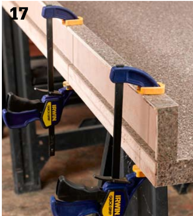
Position the backplash on the countertop, and clamp it into place with bar clamps. Wipe away the excess caulk, and let it dry completely.
