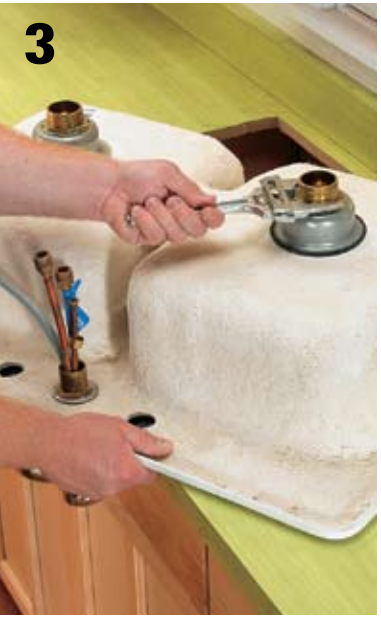
3 Attach as much of the plumbing as makes sense to install prior to setting the sink into the opening. Having access to the underside of the flange is a great help when it comes to attaching the faucet body, sprayer, and strainer, in particular.
