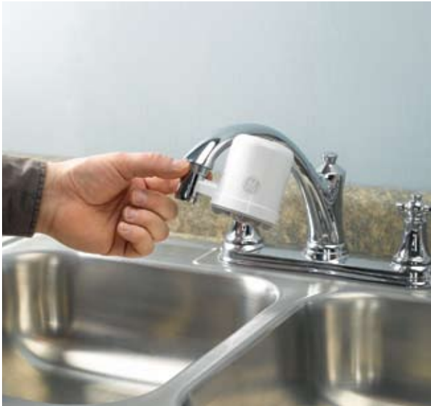
Faucet-mounted filters are the easiest to install. Remove the faucet aerator, then thread the filter unit onto the spout and hand-tighten. Slowly turn on the cold water tap, then check for leaking. If necessary, carefully tighten the collar using pliers. Flush the filter before use as recommended.
