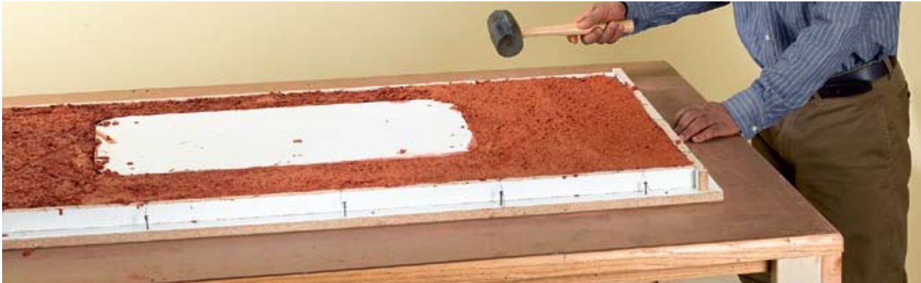
Concrete countertops are cast in forms in a well-ventilated work area and then transported to the cabinets after they are machined and polished.
