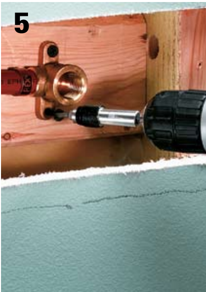
At the cooktop, install the faucet union as specified by the manufacturer. Add blocking as needed. The pot filler installed here attaches to a drop-ear L-fitting mounted to the blocking. Apply pipe joint compound to the faucet inlet and thread it onto the L-fitting.
