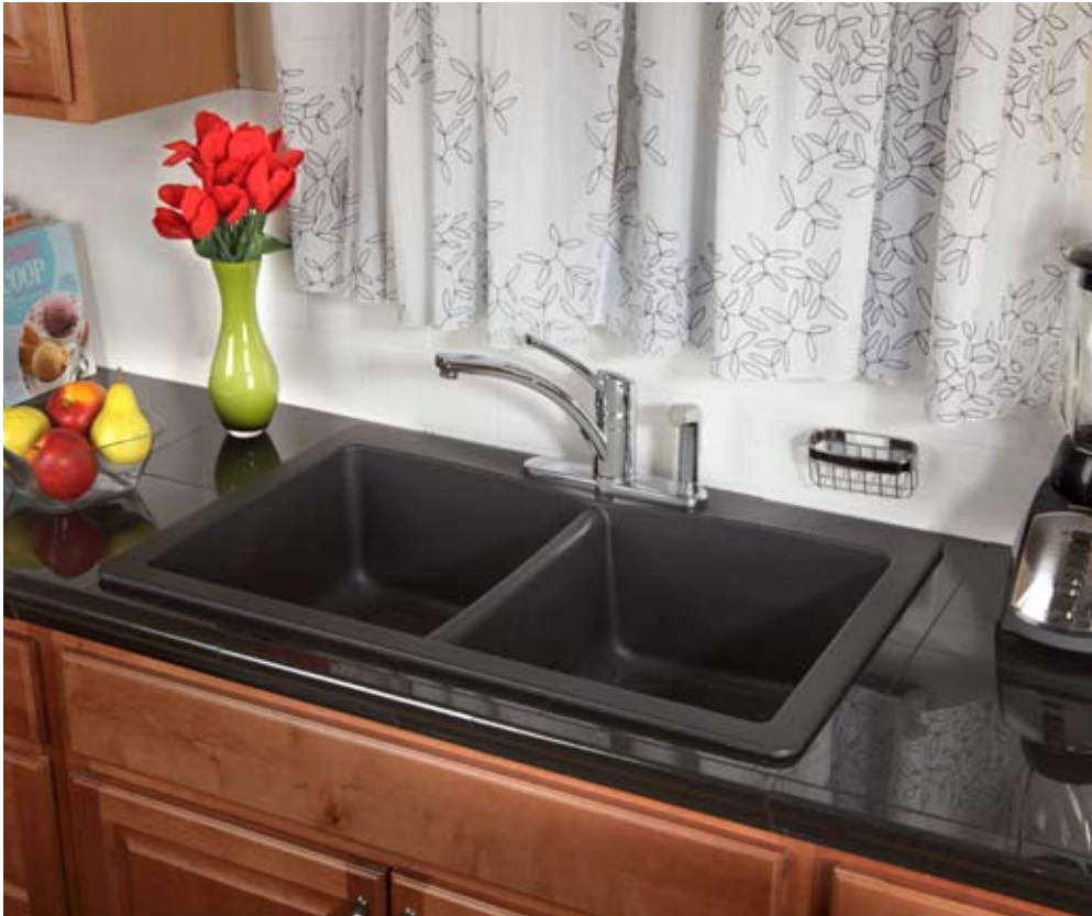
Granite tiles are installed in much the same way as ceramic tiles, but the ultra-narrow gaps and matching grout mimic the appearance of solid polished granite.
