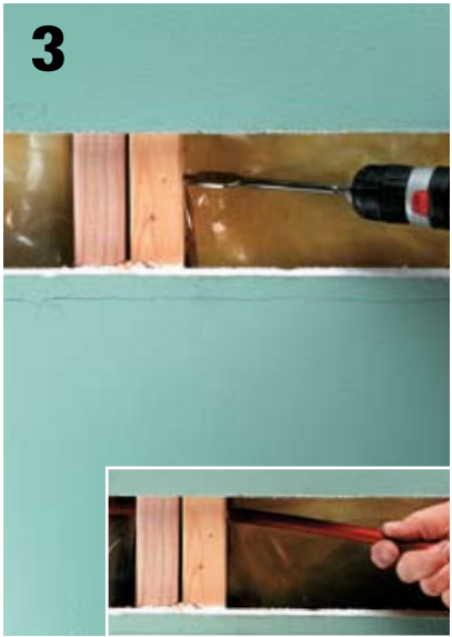
Drill 3/4" holes in the framing for the supply tubes. Install protector plates if the holes are within 1 1/4" of the stud edge. Run 1/2" PEX from the supply riser through the holes to the pot filler location (inset).
