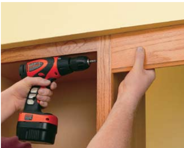
Remove valances above cabinets. Some valances are attached to the cabinets or soffits with screws. Others are nailed and must be pried loose.
