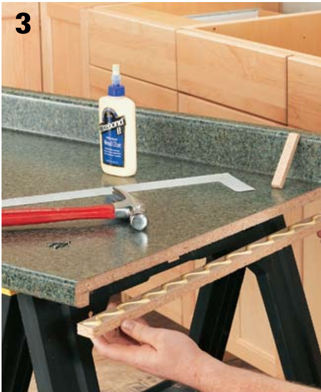
Attach the battens from the endcap kit to the edge of the countertop using carpenter's glue and small brads. Sand out any unevenness with a belt sander.
