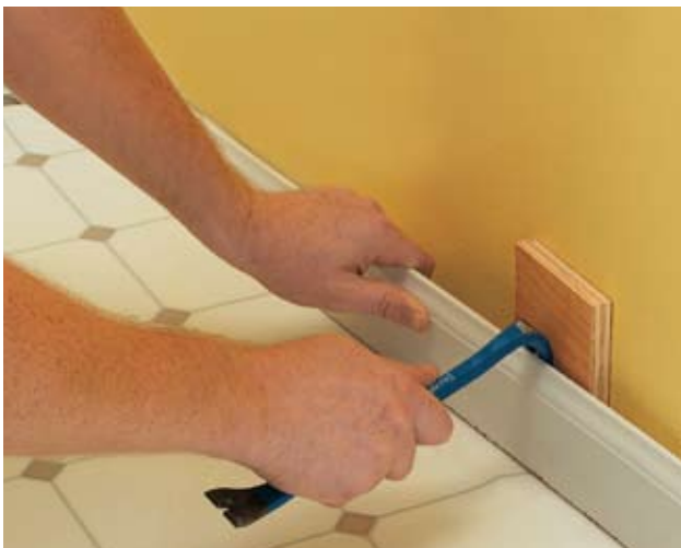
Remove baseboards and other trim moldings with a pry bar. Protect wall surfaces with scraps of wood. Label the trim boards on the back side so you can replace them correctly.
