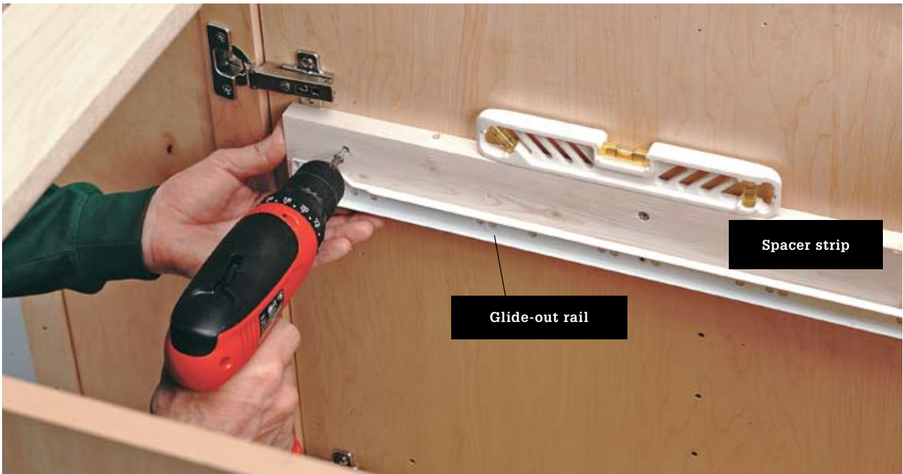
Spacers must be mounted to the wall cabinets before you can install drawer slides for your slide-out shelves. They are necessary for the drawers to clear the cabinet face frame and the door. For a ¾" spacer, a 1 × 3 or 1 × 4 works well. Paint or finish it to match the cabinet interior.
