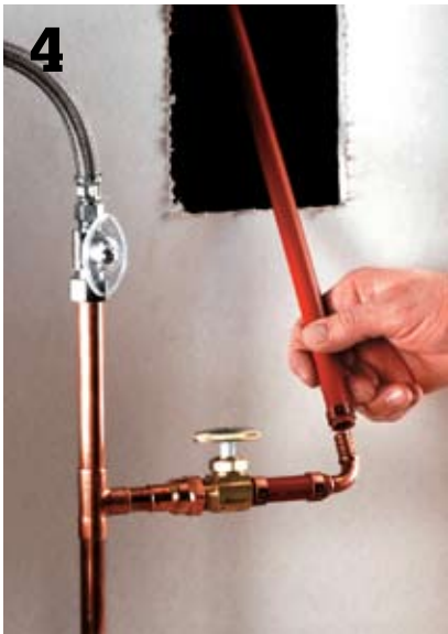
Attach the new PEX supply line to the T-fitting at the supply riser, installing an accessible shutoff valve on the new line.
