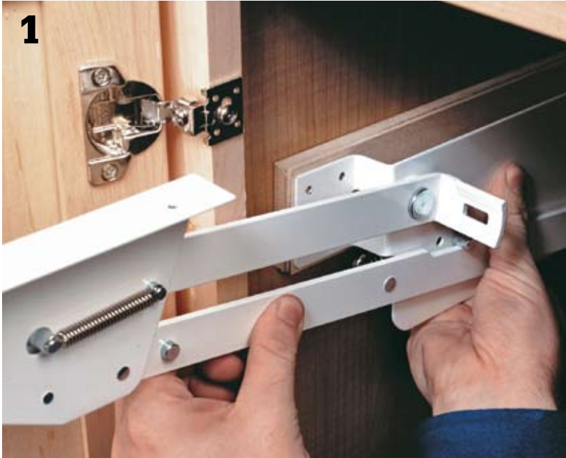
Carefully trigger the locking mechanism on each swing arm, and set the arm in its fully extended position. Hold each arm against the inside face of the cabinet side and make sure the arm will clear the door hinge and/or the cabinet face frame. If the arms do not clear, you'll need to use wood spacers to allow the arms to clear the hinges or frames by at least 1/2". In most cases, one 1 × 3 spacer for each arm will provide enough clearance. Cut the spacers so they match the length of the mounting plate on the swing arms.
