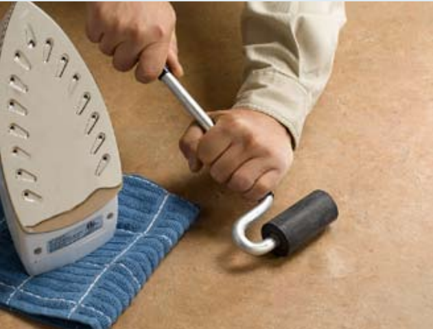
Use a J-roller to re-bond loose or bubbled laminate to its substrate. Heat the repair area with an iron first.
