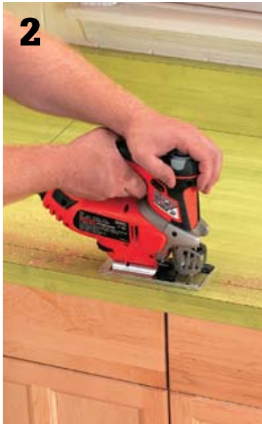
2 Drill a starter hole and cut out the sink opening with a jigsaw. Cut right up to the line. Because the sink flange fits over the edges of the cutout, the opening doesn't need to be perfect, but, as always, you should try to do a nice, neat job.
