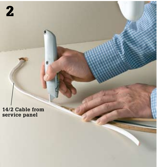
Fish a 14/2 or 12/2 cable from the electric service panel up through the hole in the floor. Strip the sheathing from the cable with a utility knife. Also strip the insulation from the wires with a wire stripper. Do not nick the wire insulation.
