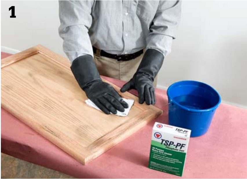
Begin painting by labeling each door and its cabinet bay with a number printed on painters' tape. This will help you replace the doors and drawers. Remove all the doors, drawers, and hardware. Clean all surfaces—front, back, top, bottom, inside, outside, edges—with a grease-cutting cleaner such as synthetic trisodium phosphate (TSP). Follow the directions carefully.
