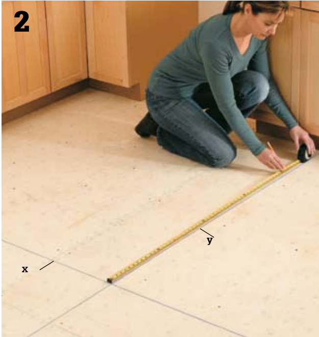
Check the reference lines for squareness using the 3-4-5 triangle method. Measure along reference line X and make a mark 3 ft. from the centerpoint. Measure from the centerpoint along reference line Y and make a mark at 4 ft.
