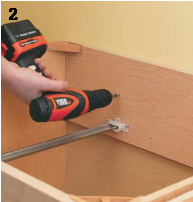
2 At the backs of cabinets , remove any screws holding the cabinet to the wall. Cabinets can be removed as a group or can be disassembled.
