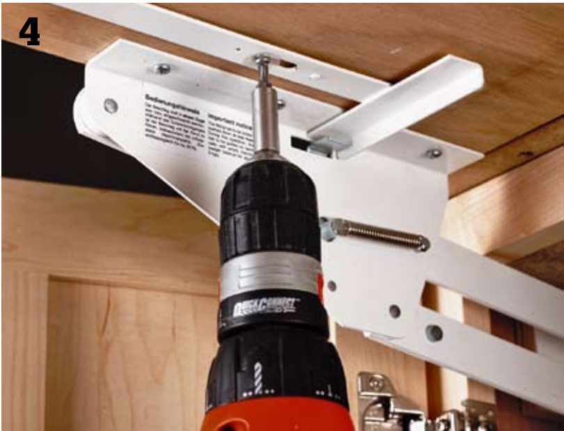
Fasten each locking bar to the bottom shelf face with the provided screws and plastic spacers to ensure the bars will slide smoothly. Test the locking bars' operation with the shelf in the extended and retracted positions, and make any necessary adjustments.
