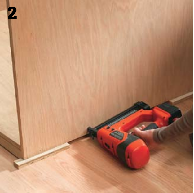
Cut the bottom panels the same dimensions as the base frame from ¾" birch plywood. Attach it to the frame with finish nails. Then, cut the side panels to size and shape and fasten them to the edges with 6d finish nails and adhesive. Slip ¾" shims (scrap plywood works well) beneath the side panels before fastening them.
