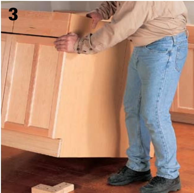
Join the two base cabinets together by driving 1¼" wallboard screws through the nailing strips on the backs of the cabinets from each direction. Make sure the cabinet sides are flush and aligned. Lower the base cabinets over the cleats. Check the cabinets for level, and shim underneath the edges of the base if necessary.
