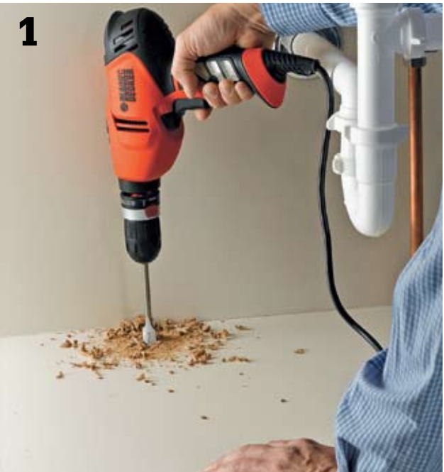
Drill an access hole for a new power cable (in flexible conduit) in the bottom of the sink compartment cabinet. Use a drill and a 3/4"-dia. bit. Go into the basement and drill a hole up through the flooring that will align with the first hole or make other arrangements to run circuit wire.
