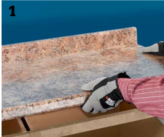
1 Remove the countertops. From inside the base cabinets, unscrew the screws holding the countertops to the cabinets. Unscrew take-up bolts on mitered sections of the countertop. Use a utility knife to cut through the caulk, if present. Countertops should lift off easily, but if they don't, you can use a prybar to carefully pry them away from the base cabinets. Note: In some cases you can install these tiles over old laminate countertops (see previous page).
