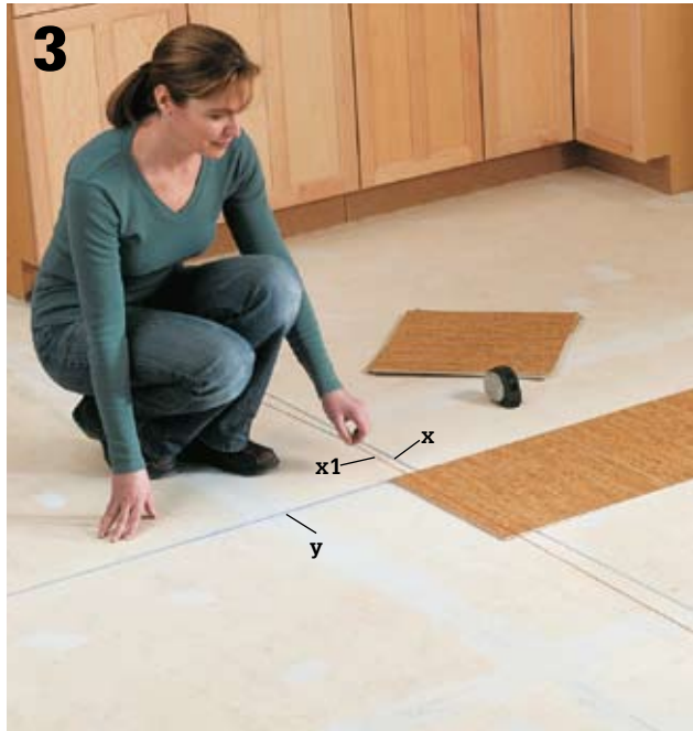
Create a new line that is parallel to reference line X and runs through a tile joint near line X if it's necessary to shift the layout. The new line, X1, is the line you'll use when installing the tile. Use a different colored chalk to distinguish between lines.
