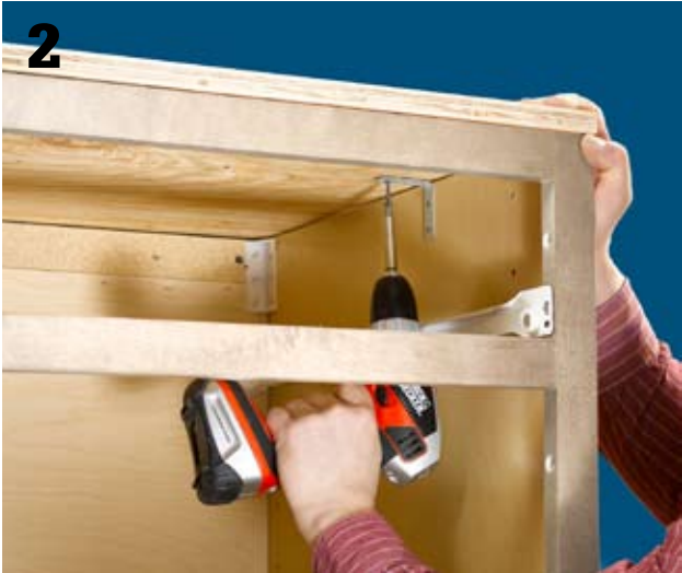
2 Prepare and install the subbase. Measure the cabinet bank from outside edges to outside edges on all sides and cut a piece of 5/8"-thick exterior grade plywood to fit. The edges of the plywood should be flush with the outside edges of the cabinet tops. Screw the plywood to the cabinet braces from underneath.
