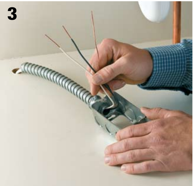
Slide a piece of flexible conduit over the wires, so the wires are protected from the point where they leave the cabinet floor to where they enter the electrical box. Attach the conduit to the box with a box connector so at least 8" of wire reaches into the box.
