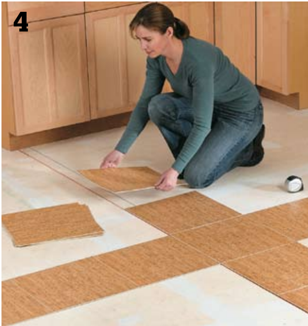
Dry-fit tiles along the new line, X1. If necessary, adjust the layout line as in steps 1 and 2.
