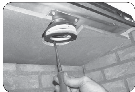
Fig. 56-4 Install plate and gaskets
