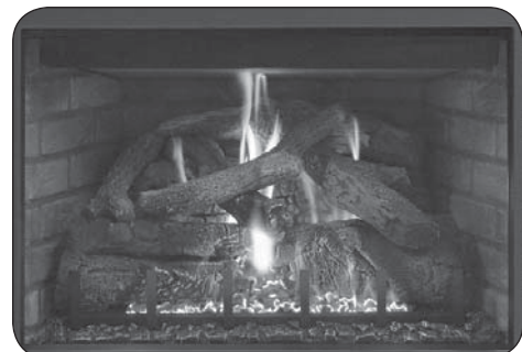
Fig. 54-5 Proper flame appearance
