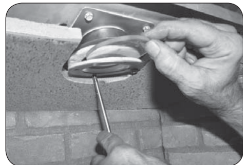
Fig. 56-5 Install glass & fasten all screws
