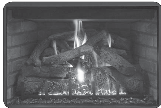
Fig. 53-2 Proper flame appearance
