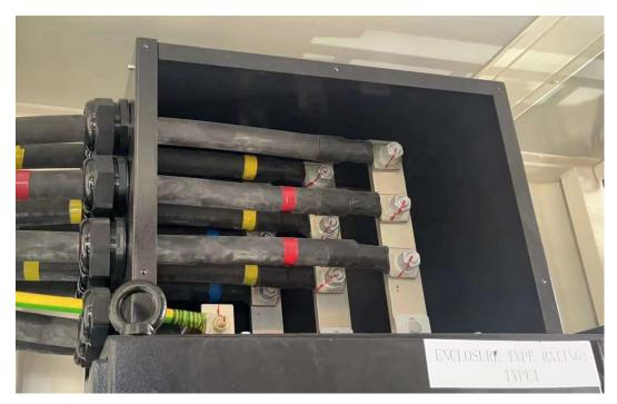
Figure 8-20 Cable connection diagram
