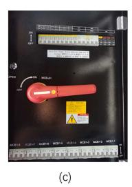
Figure 8-2 (a) Distribution cabinet circuit breakers (b)Internal of the main control cabinet (c)The main circuit breaker of the distribution cabinet
