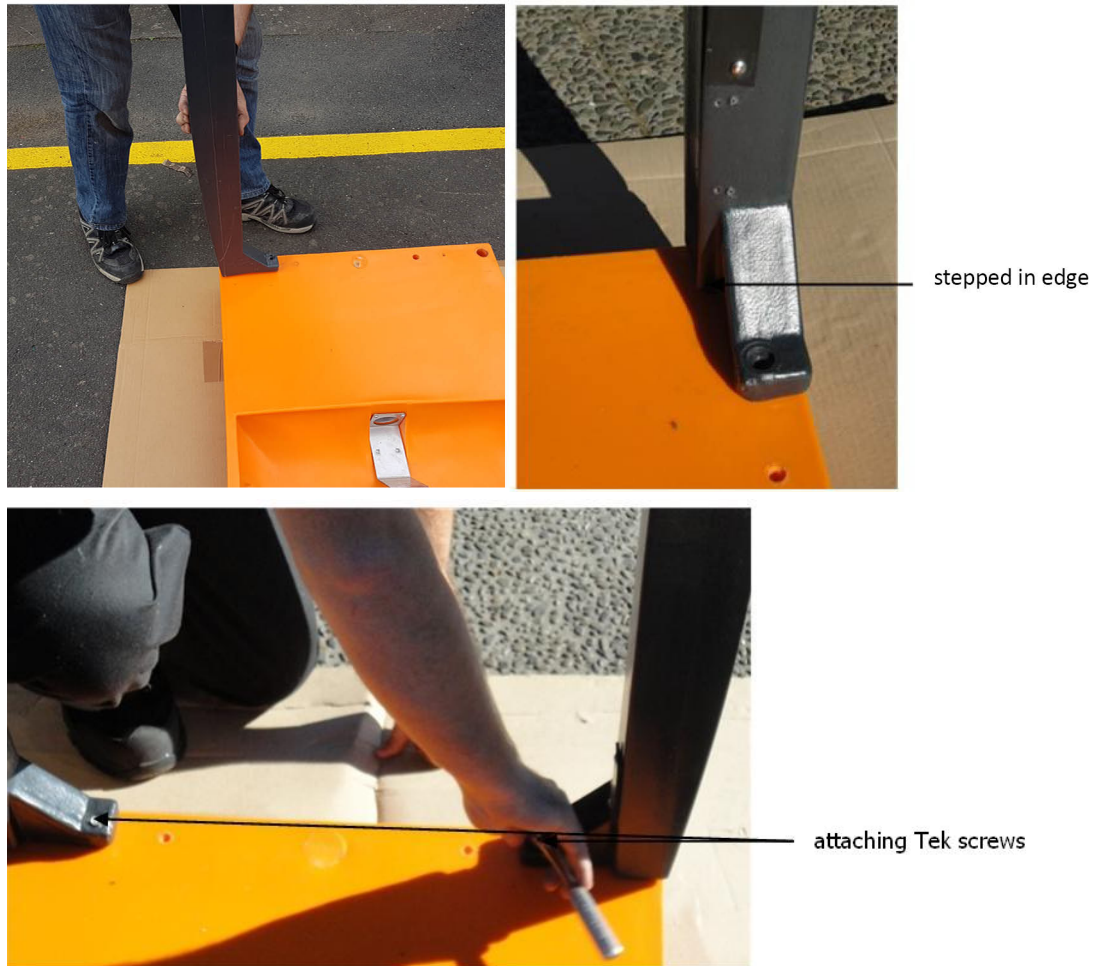
Figure 11. Roof tie bar assembly
