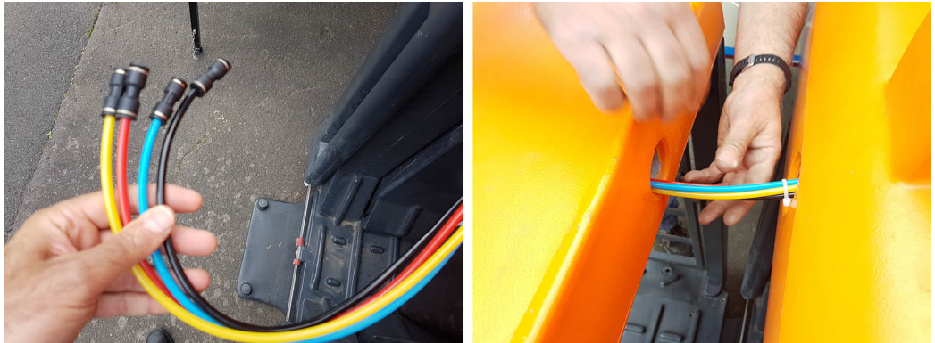
Figure 16. Inserting air lines.
