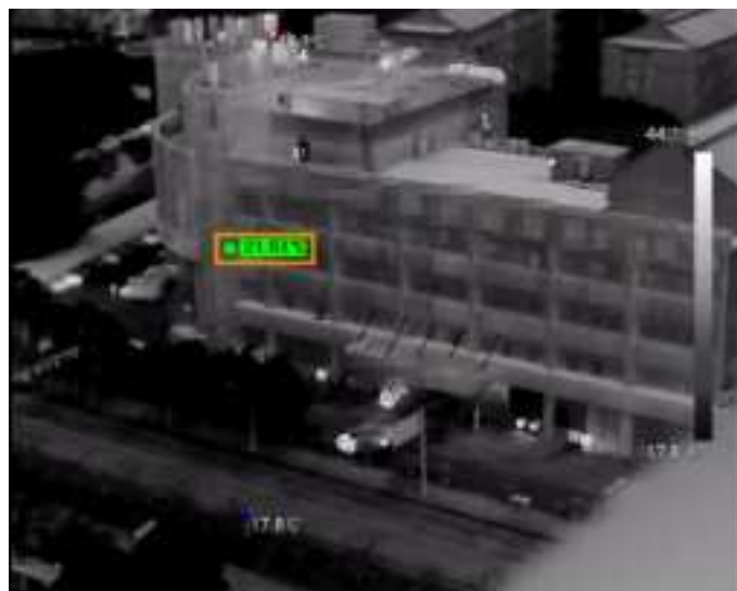
Figure 4-6 Real-time spot temperature measurement
