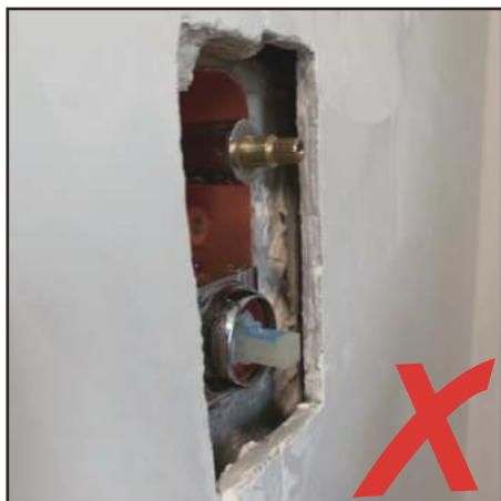
Valve installed too deep- incorrect installation
