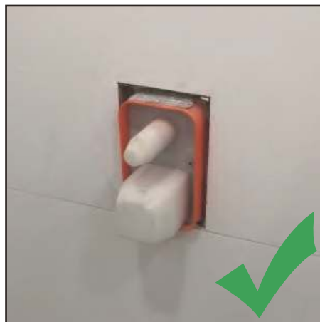
Correct installation
