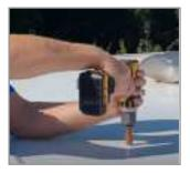
Check the hole is straight by drilling one last time from inside.
