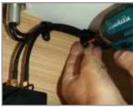
Connect the 12V DC Power to the Power input and then screw the two SMA cables from the antenna to the SMA Inputs on the docking station (These can go either way around, there is no sepcific SMA port to a cable).
