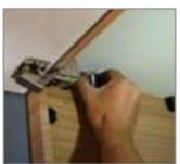
With the remaining adhesive, apply a fine bead around the antenna base to seal the antenna installation and allow to dry.
