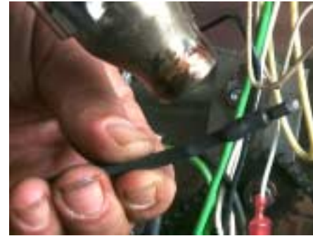
Fig: 16 Use a heat gun to secure the shrink wrap in place..
