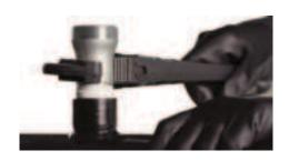
4. Use a pipe wrench to connect the flexible hose to the inlet nipple. Torque range should be a minimum of 50 to a maximum of 58 ft-lbs.
