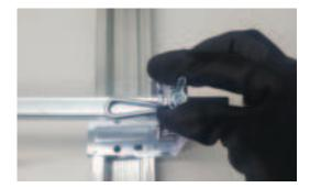
8. Tighten two sheet metal screws on each end of the bracket, making sure to fully penetrate the hat furring channel. The recommended torque is 1.40–1.48 ft-lbs (190-200 cN • m).
