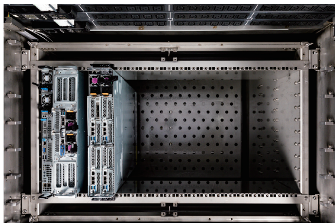
▲ Overhead view of A1P0-EB0 Tank
