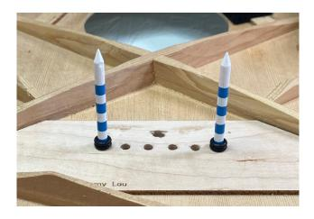
Install the golf tees in the two outer endpin holes, and slide two of the supplied small rubber grommets over each golf tee on the inside of the guitar as shown. These will hold the tees firmly in place, and they also serve as a spacer between the cardboard template and the bridgeplate so it won't stick to the E6000 cement during installation.
