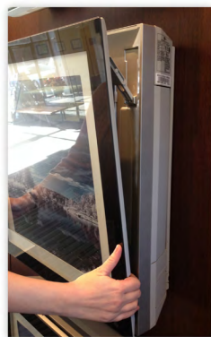
2. Pull front panel away at the bottom.
