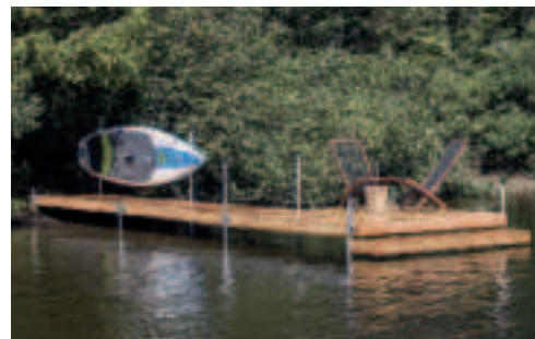
Make small stationary dock sections to ease winter removal
