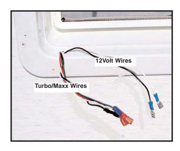
14. Connect the four wires from the Turbo/Maxx power cable to the PC board in the control box. These terminals marked FAN are located near the center of the board. Push the white wire (smaller female terminal) onto the horizontal male terminal labeled WHITE COM. Connect the green wire to the horizontal male terminal labeled GREEN LOW, the red wire to the horizontal male terminal labeled RED MED and the black wire to the horizontal male terminal labeled BLACK HIGH. (I)
