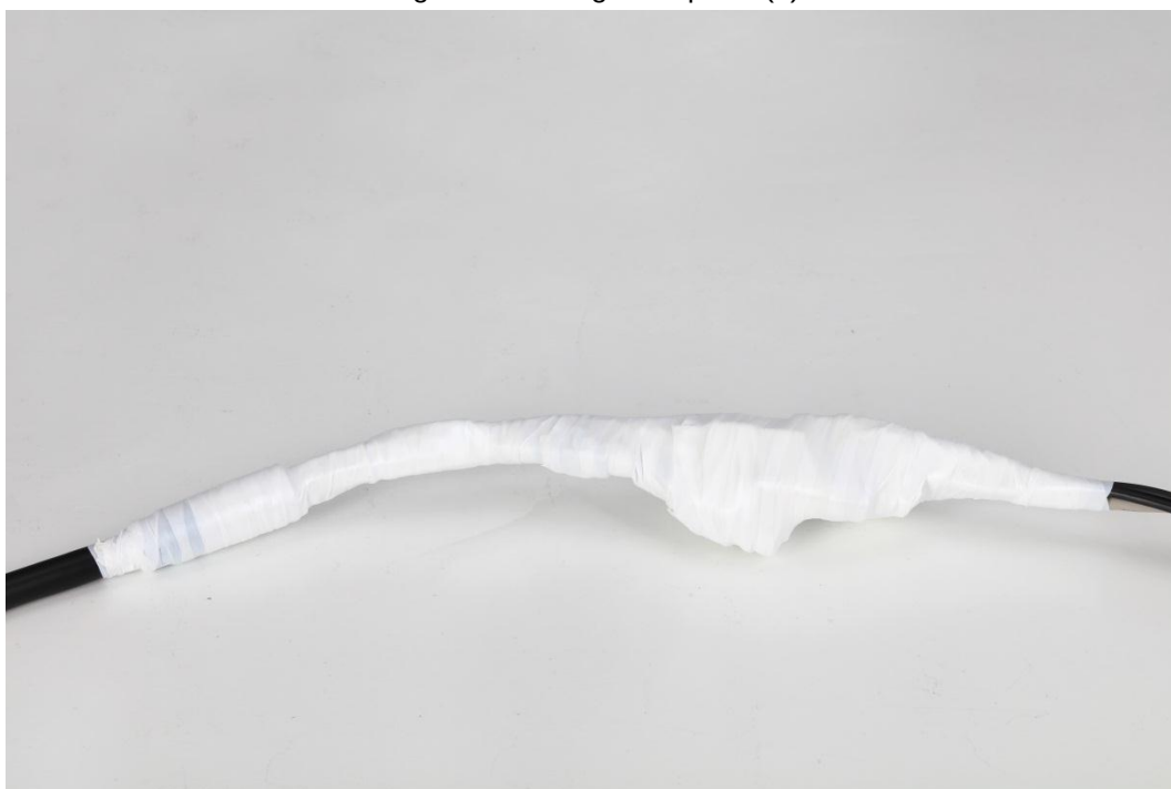
Figure 1-5 Doing waterproof (2)
