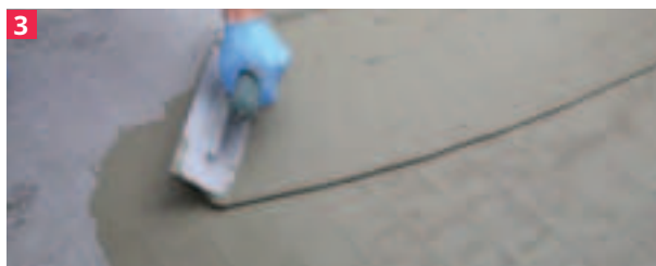
Trowel thinset and install tile
