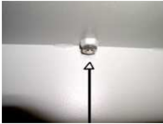
Fig. 4: Counter nut
