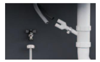
1. Turn off the water supply. Disconnect the drain hoses from the sink drain pipe, and disconnect the water inlet pipe from the water valve.
