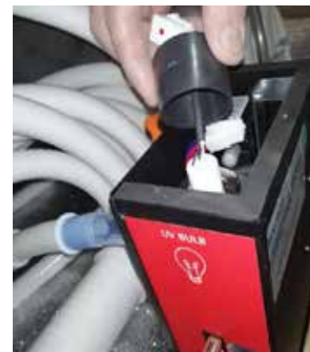
Step 4: Take out this black protective sleeve
