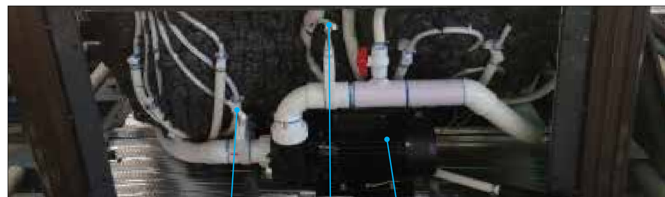
Slice valve Slice valve Pump
