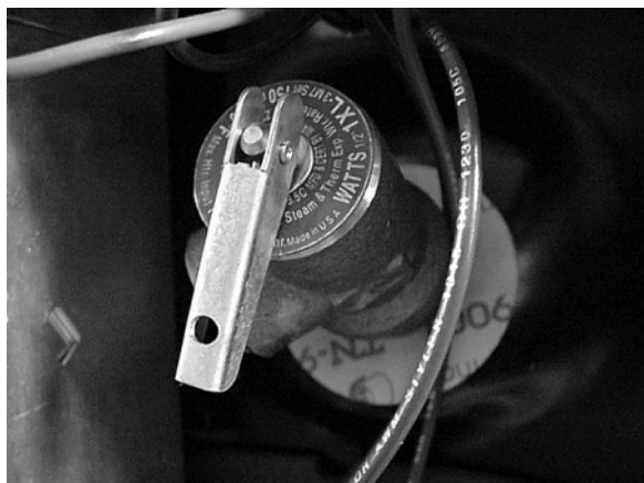
Lift straight out to open P-T valve
