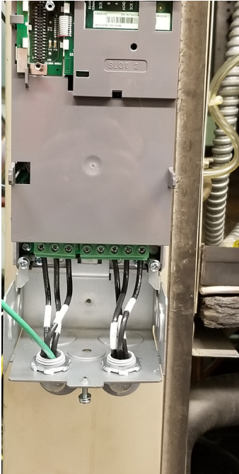
Figure 13: Actuators for Waterside Economizer
