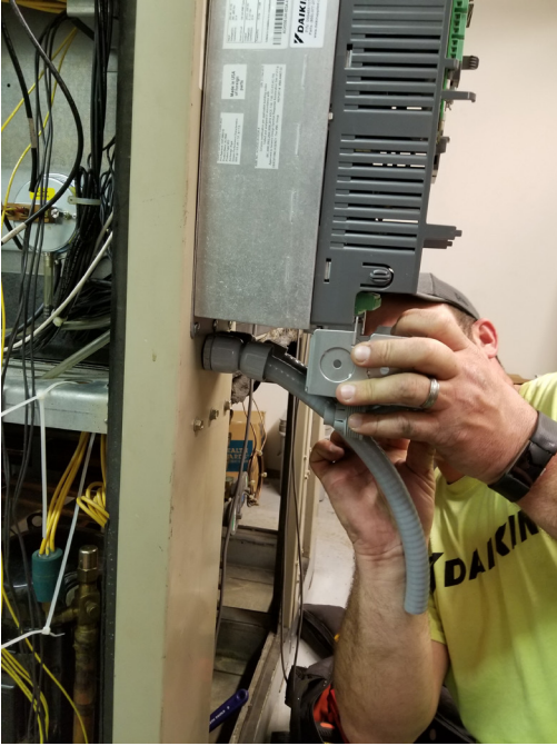
Figure 12: Actuators for Waterside Economizer
