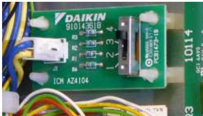
Figure 45: 4-Position Fan Speed Selector Switch
