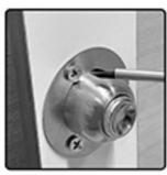
STEP3: Install 3 screws to fix the base
