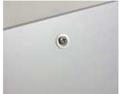
Install washer between screw and shelf
