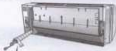
Shape the connection pipe
