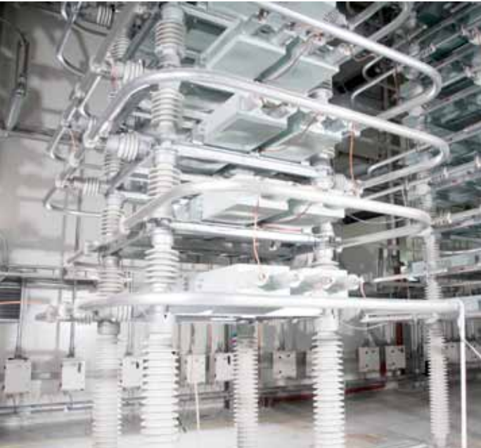
Capacitor bank for test room
