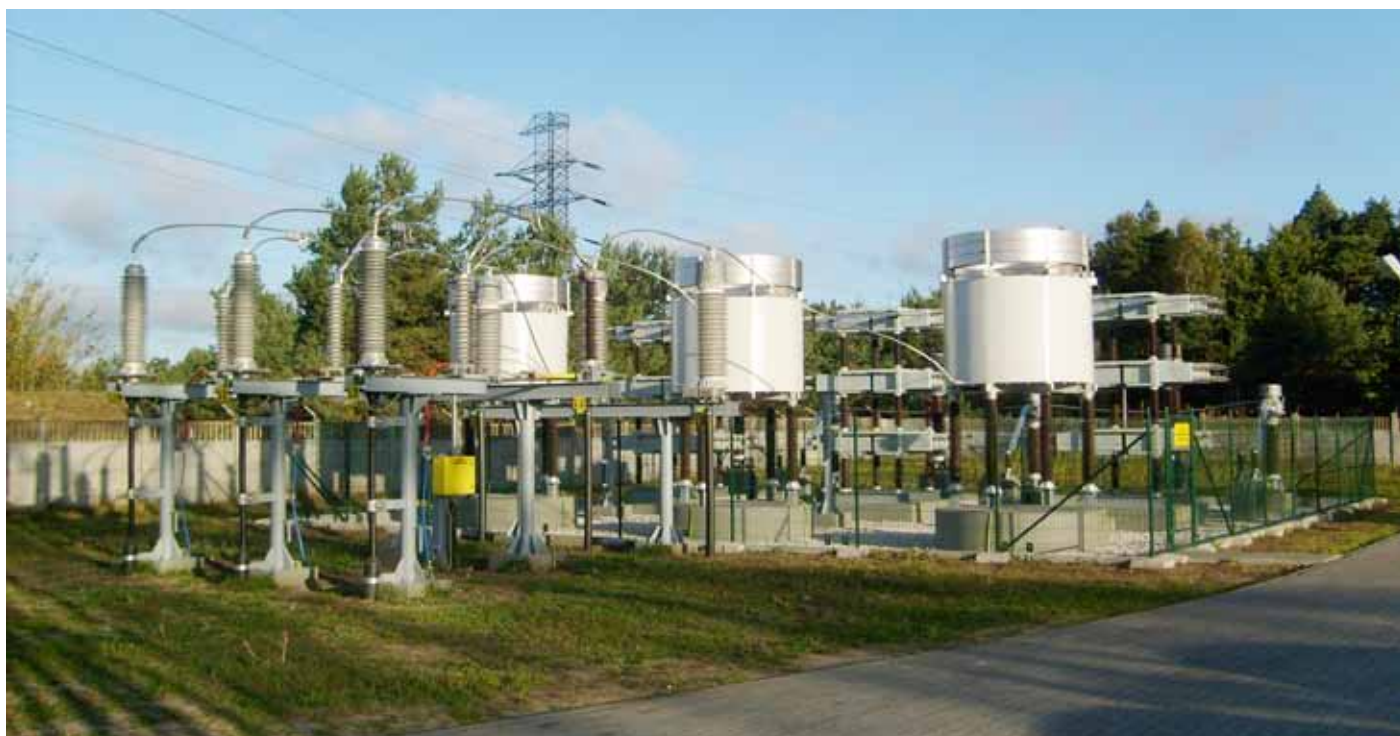
110 kV/50 Mvar filter installation at PSE substation in Poland
