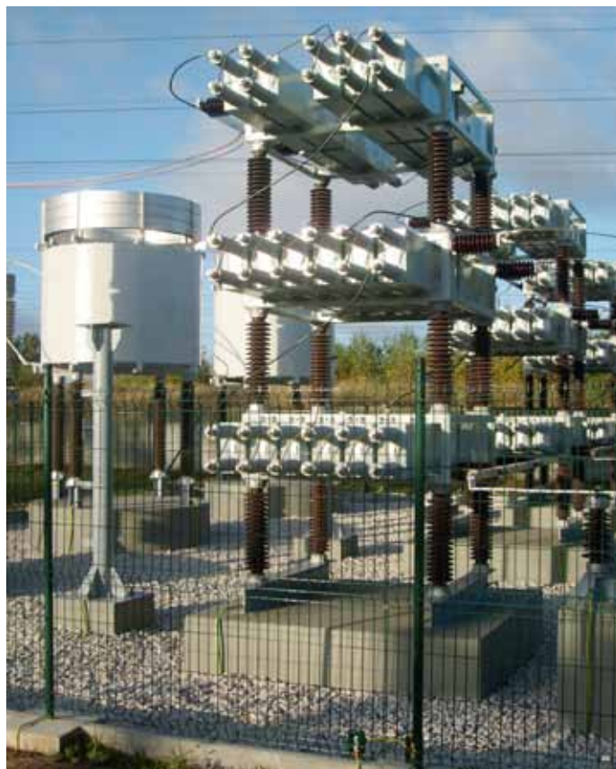
110 kV/50 Mvar filter installation at PSE substation in Poland
