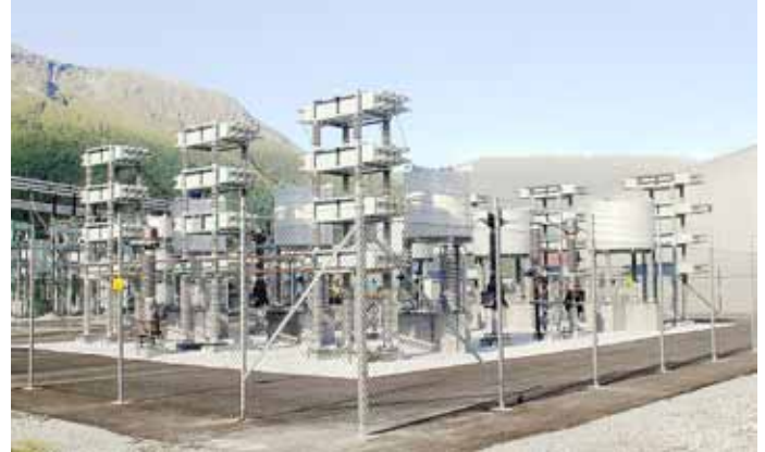
145 kV filter installation in Norway.
