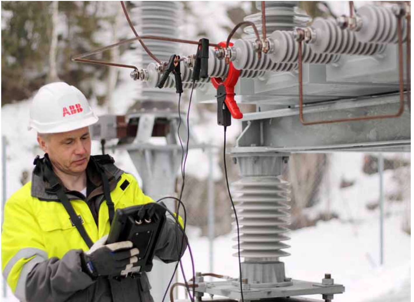
Measuring of capacitance in capacitor bank, Norway
