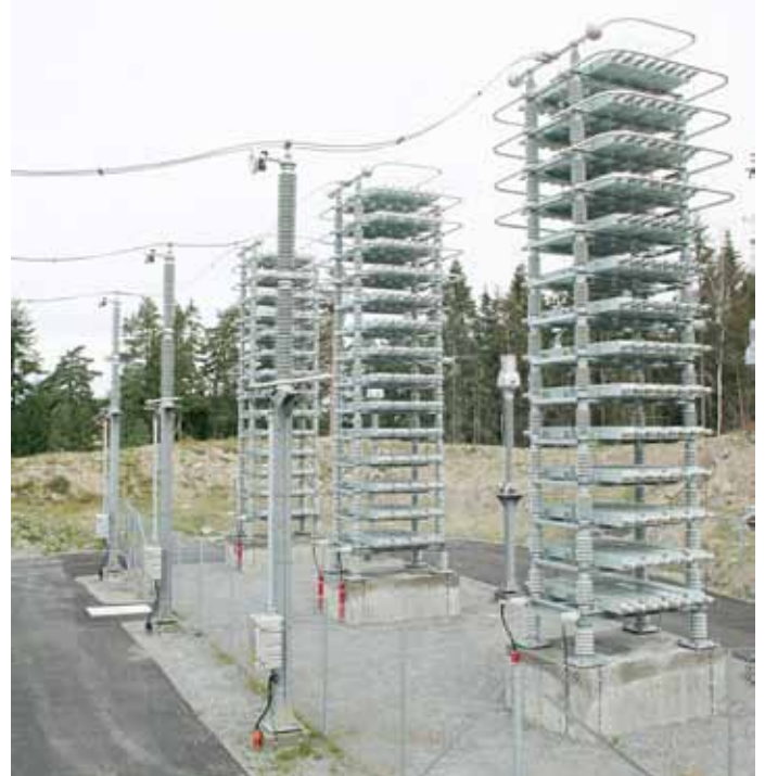
420 kV capacitor bank installation in Norway.
