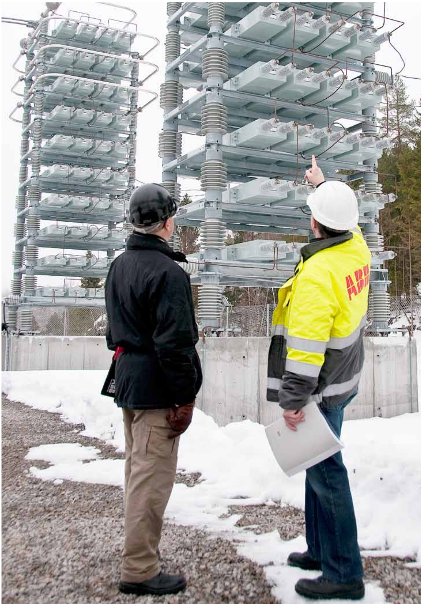
300 Mvar/420 kV/50 Hz capacitor installation in Norway
