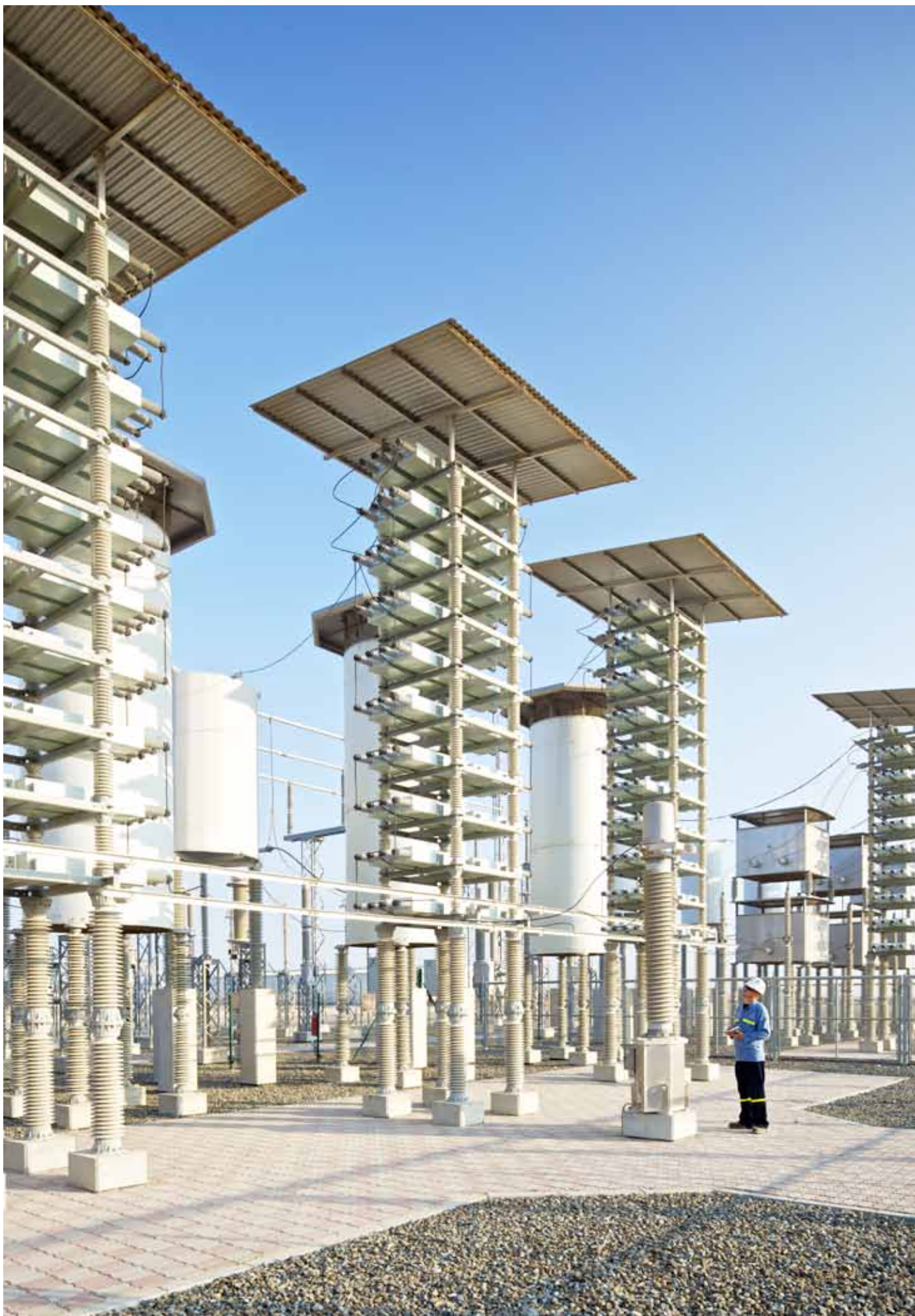
145 kV filter installation in Oman
