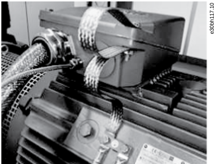
Illustration 2: Installation of EMC straps from the Terminal Box to the Motor Frame
