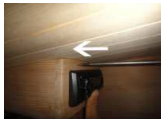
FIG-15.4 Screw wood housing to sauna room
