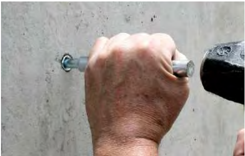
Anchor being set with hand setting tool.
