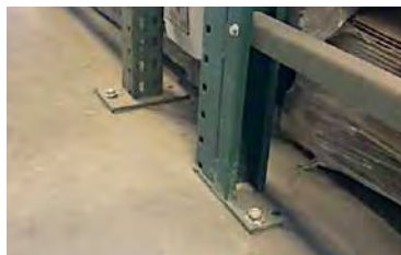
Typical low-corrosive environment — interior warehouse.
