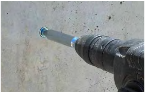
Anchor being set with SDS setting tool.
