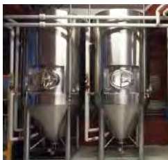
Typical high-corrosive environment — food-processing plants.
