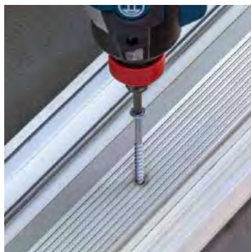
Sliding door track installation
