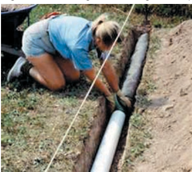
Figure 271:Underground Refrigerant Piping.
