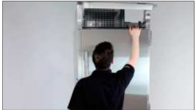
FIG. 3. Be sure to inspect behind the rainshield.
