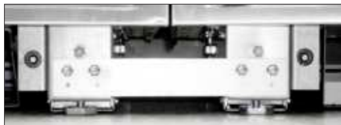
FIG. 18. Installed joining bracket.
