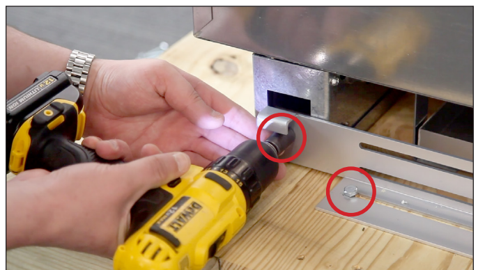
FIG. 8. Anti-tip bracket shipping bolt locations. Other side not shown.
