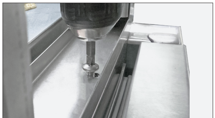
FIG. 10. Remove the screws from the metal channel.
