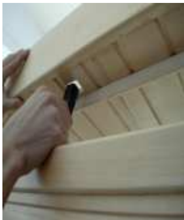
FIG-12 Slip cords/wires through corresponding holes
