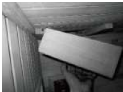
FIG-16 Installing the Radio Wood Housing
