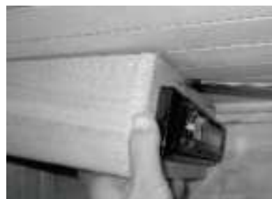
FIG-17 Screwing in the Radio Wood Housing
