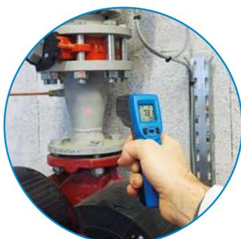
VERIFICA TEMPERATURE IN ENTRATA E IN USCITA PER IMPIANTI DI ACQUA CALDA SANITARIA
