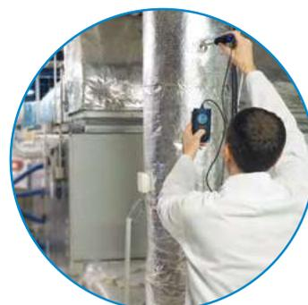
MISURARE LA VELOCITÀ DELL'ARIA, LA PORTATA E LA TEMPERATURA IN UN CONDOTTO
