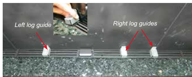
Log guides installed
