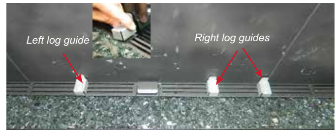
Log guides installed
