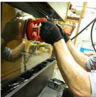
Handle glass with supplied vacuum clamps
