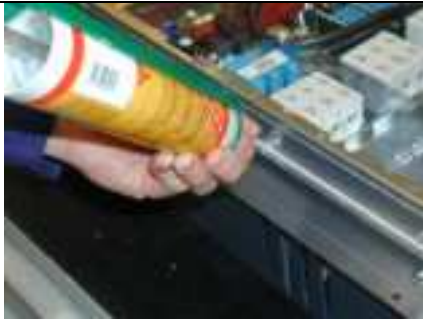
7. Seal the sides of the frequency converter.
