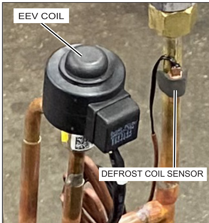
FIGURE 21. Defrost Coil Sensor Location
