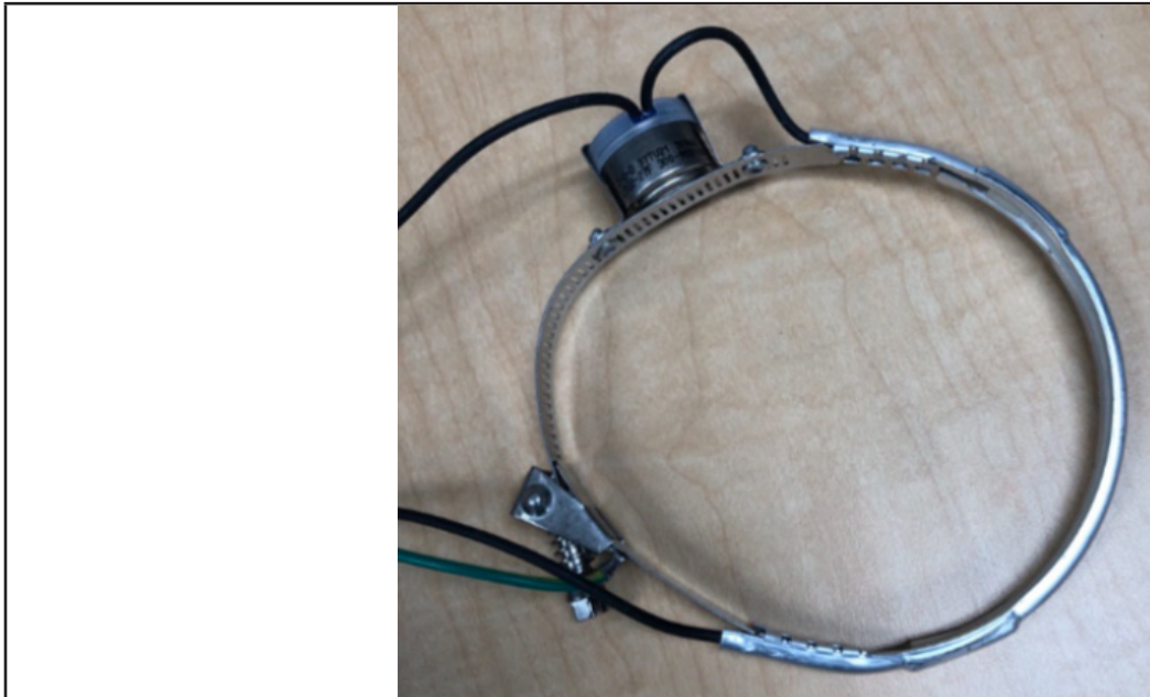
FIGURE 36. Belly-Band Crankcase Heater Thermostat
