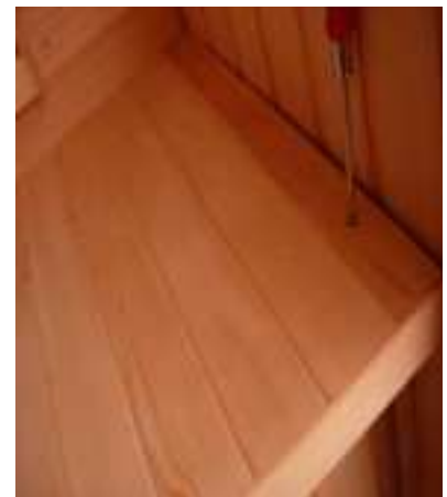
FIG-10 Securing Benches with screws
