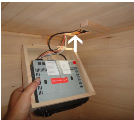
FIG-15.3 Feed the wires up through the roof
