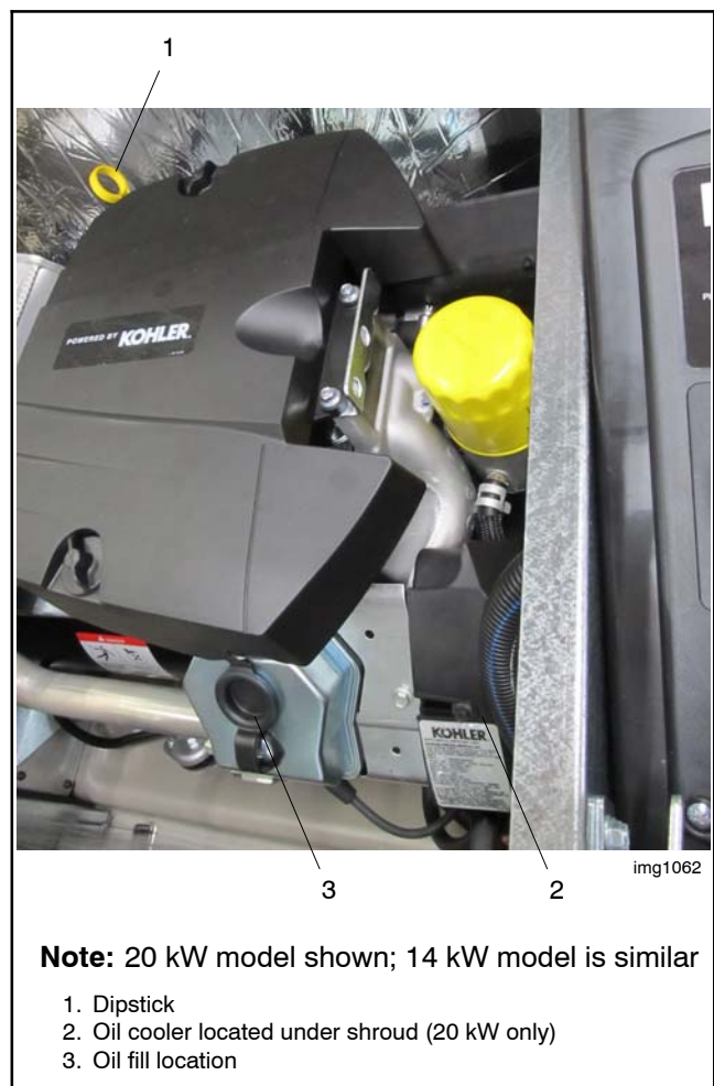
Figure 4-3 Oil Fill Components
