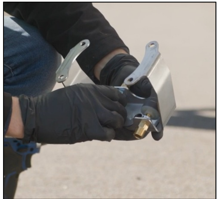
Figure 4: Install cap sensors on Flow-Thru Brackets.
