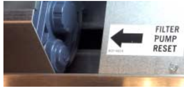
Reset switch location: New-style FPIII
