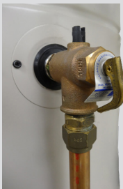
TPR position - top of cylinder
